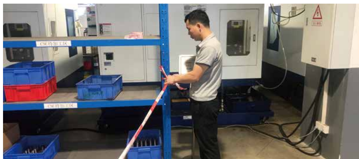
▲ Warning lines for the leaking area
