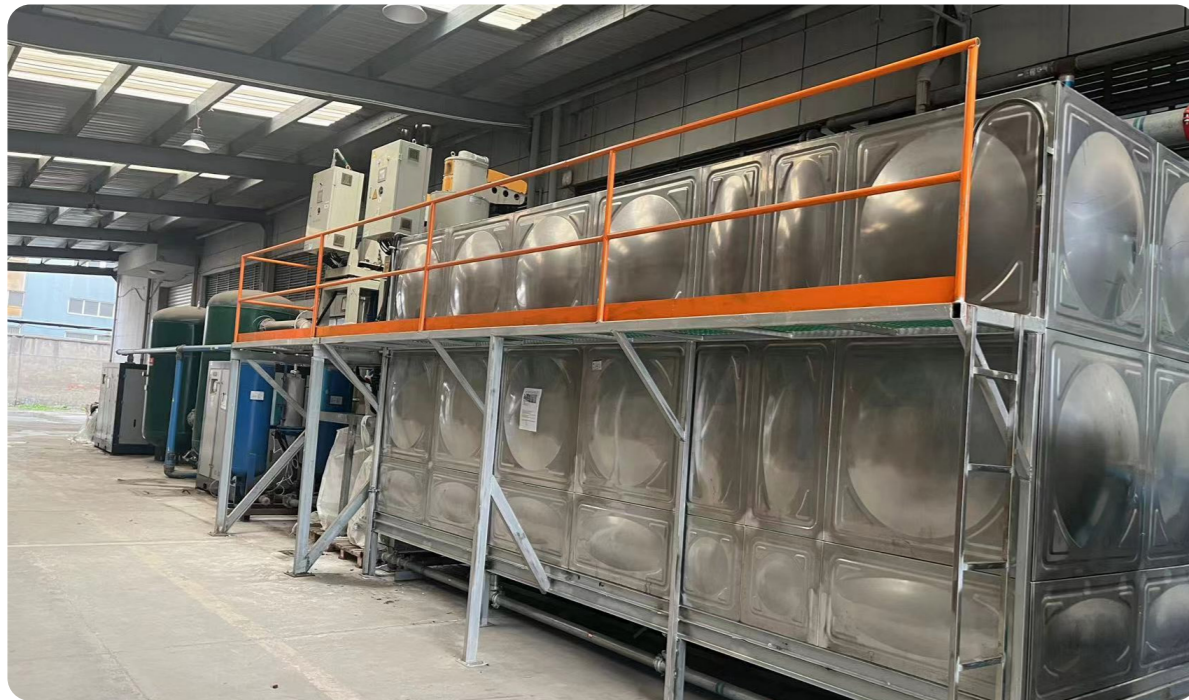
► A Glimpse of the Centralized Water Supply for Precision Carving Machines at the Second Branch of Goneo Electric
