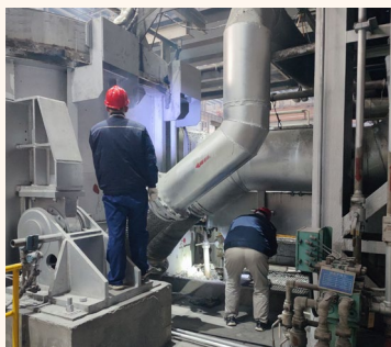
Special Inspection of Deep Well Casting in the Flat-Rolled Product Division
