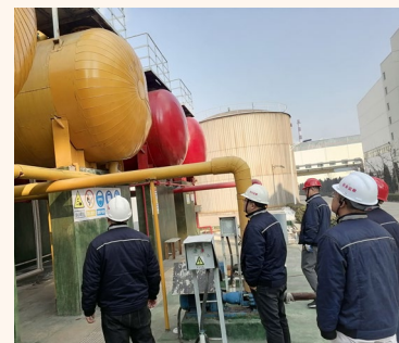
Hazardous Chemicals Special Inspection of Donghai Power Plant
