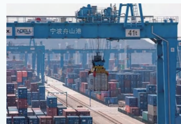
Completed the automation transformation of 16 rail-mounted cranes, achieving full automation of the existing 52 rail-mounted cranes.
