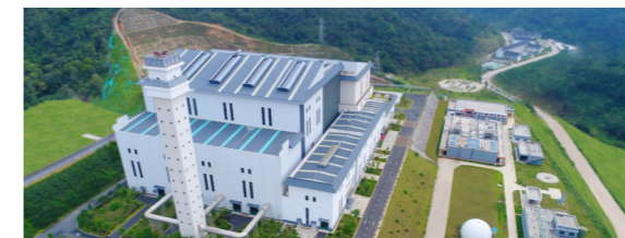
the Municipal Solid Waste Incineration Flagship Project - Huizhou Waste-to-Energy Project in Guangdong Province
