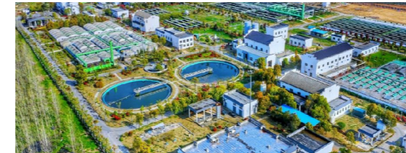
the Sewage Treatment Flagship Project - Hefei Shiwuli River Sewage Treatment Project in Anhui Province
