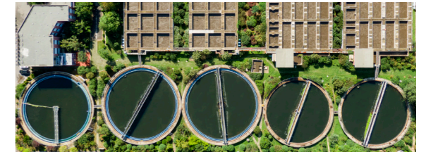
the Recycled Water Service Flagship Project - Dalian Hengji Recycled Water Project in Liaoning Province
